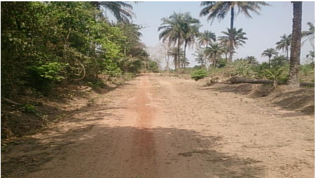
Road Constructed by Miro Forestry SL Ltd leading to Petifumayagbo, Foindu Section, Yoni Chiefdom
