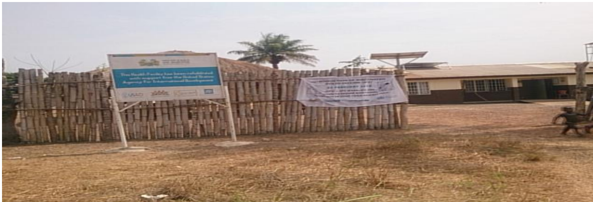
Health Center constructed by Government of Sierra Leone at Patfumayagbo Foindu Section, Yoni Chiefdom
