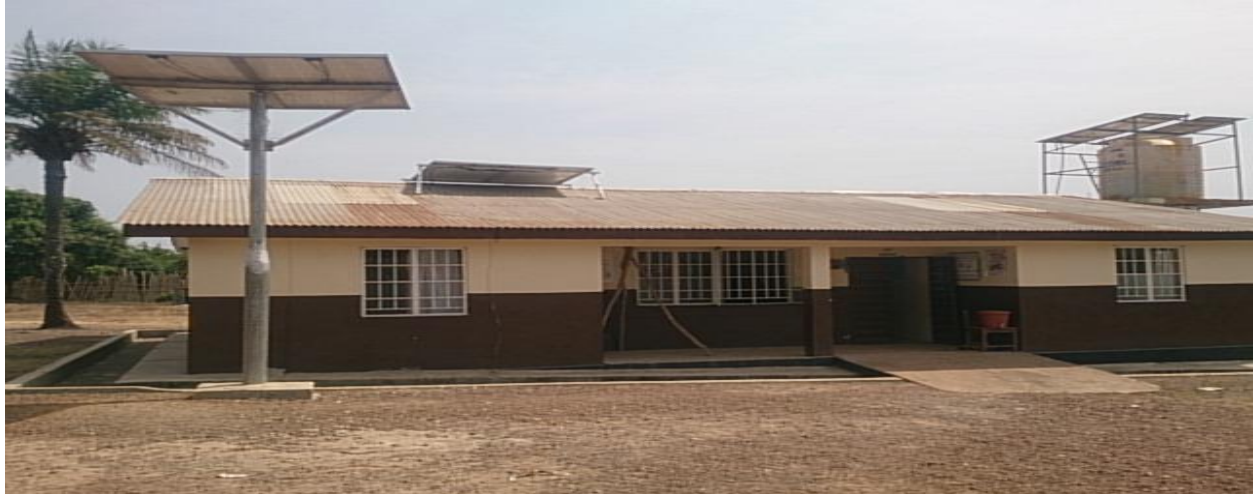
Health Center constructed by the Government of Sierra Leone at Patfumayagbo Foindu Section, Yoni Chiefdom
